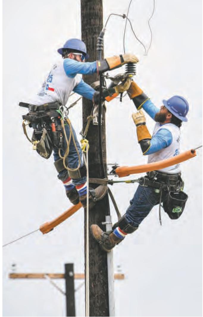
Journeymen Ty Duesterheft and John Zamora from Maxwell change out power line equipment during the 2025 Texas Lineman's Rodeo.
